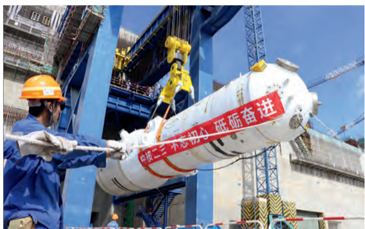
“华龙一号”全球首堆蒸发器吊装
